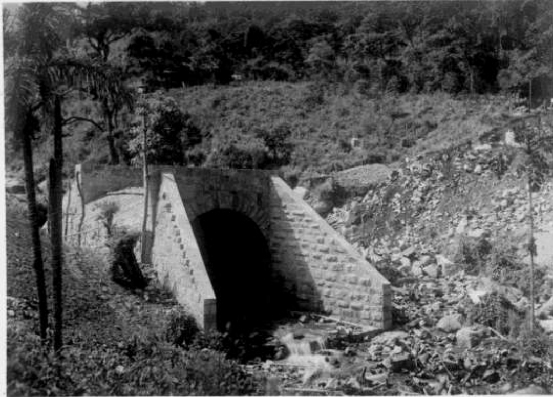
Obra # 149, Km 92+140.50, Serv. Rural, Grm. Quebr. Cajón
